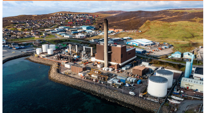
Shetland Grid Supply Point - an SSEN Distribution project under construction
