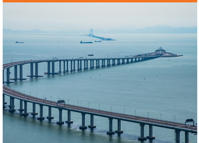
BASEC approved Firecel cables installed into the Hong-Kong-Zhuhai-Macaus Bridge
