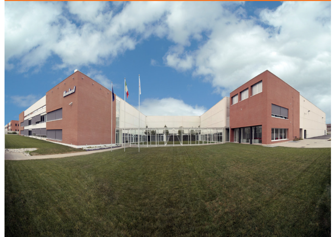
CaviceL headquarters, Milan, Italy
